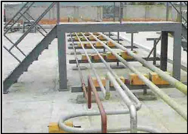
LNG – liquified natural gas receiving station cold preservation pipe support.
